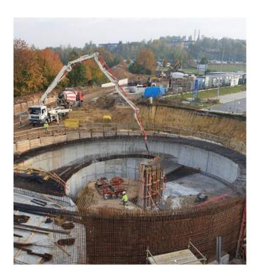
Xypex Admix C-1000 NF was selected and used for its unparalleled advantages, such as being added to the concrete during batching, eliminating the need for post-curing waterproofing membranes or coatings. The use of Xypex Admix saves time and money, renders the concrete impermeable to water, and chemically resistant. This ensures long-term durability and protection for the campus's concrete infrastructure.
